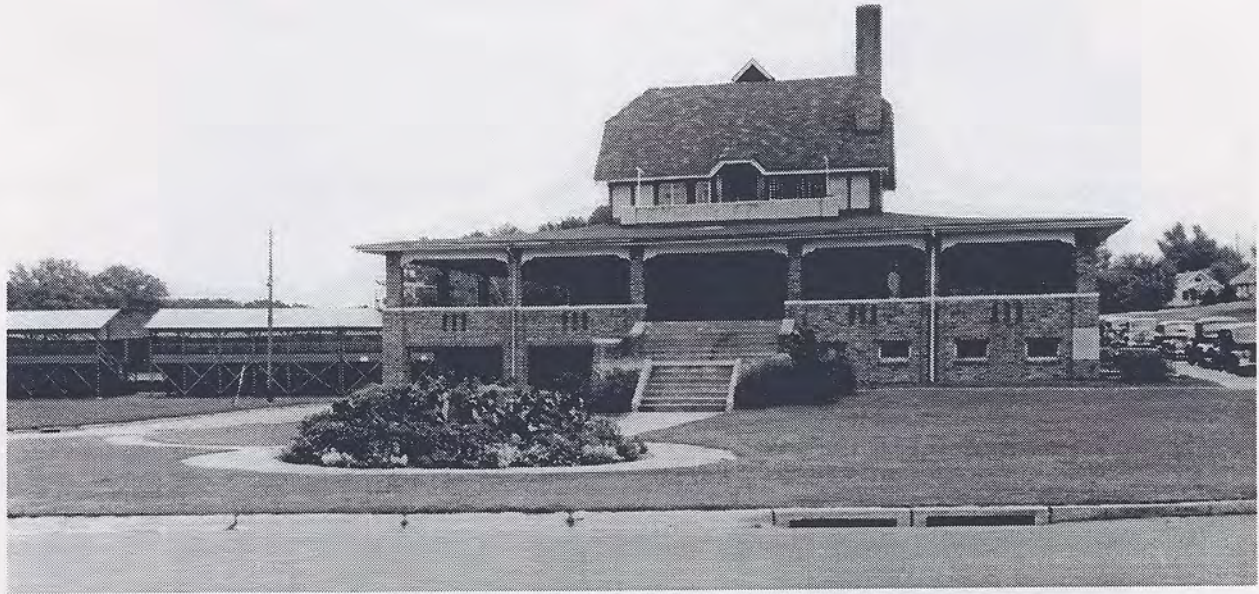
August 30, 1942, Fontenelle Park Pavilion: Photo shows new roof of the baseball grandstand at left.
